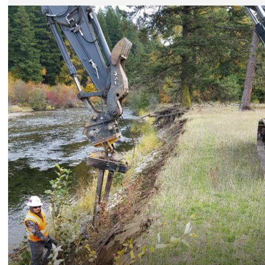
Hydraulic ram mounted on an excavator installing 5-10 ft tall riparian plants on an 8 ft terrace bank along the upper Yakima River. Photo Credit: Katrina Strathmann
